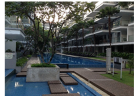
Condominiums in Singapore usually come with large sized outdoor swimming pools.
