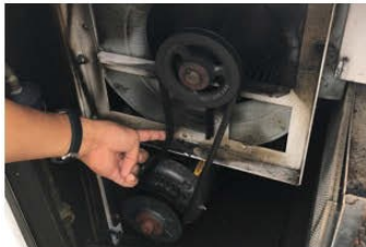
CDR Gumapas fixing a belt on a 12 ton transportable HVAC in Aguadilla, PR BoO
