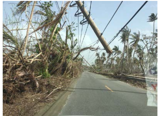
Example of damage from Hurricane
