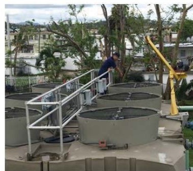
CDR Gumapas assessing a cooling tower in Bayamon, PR
