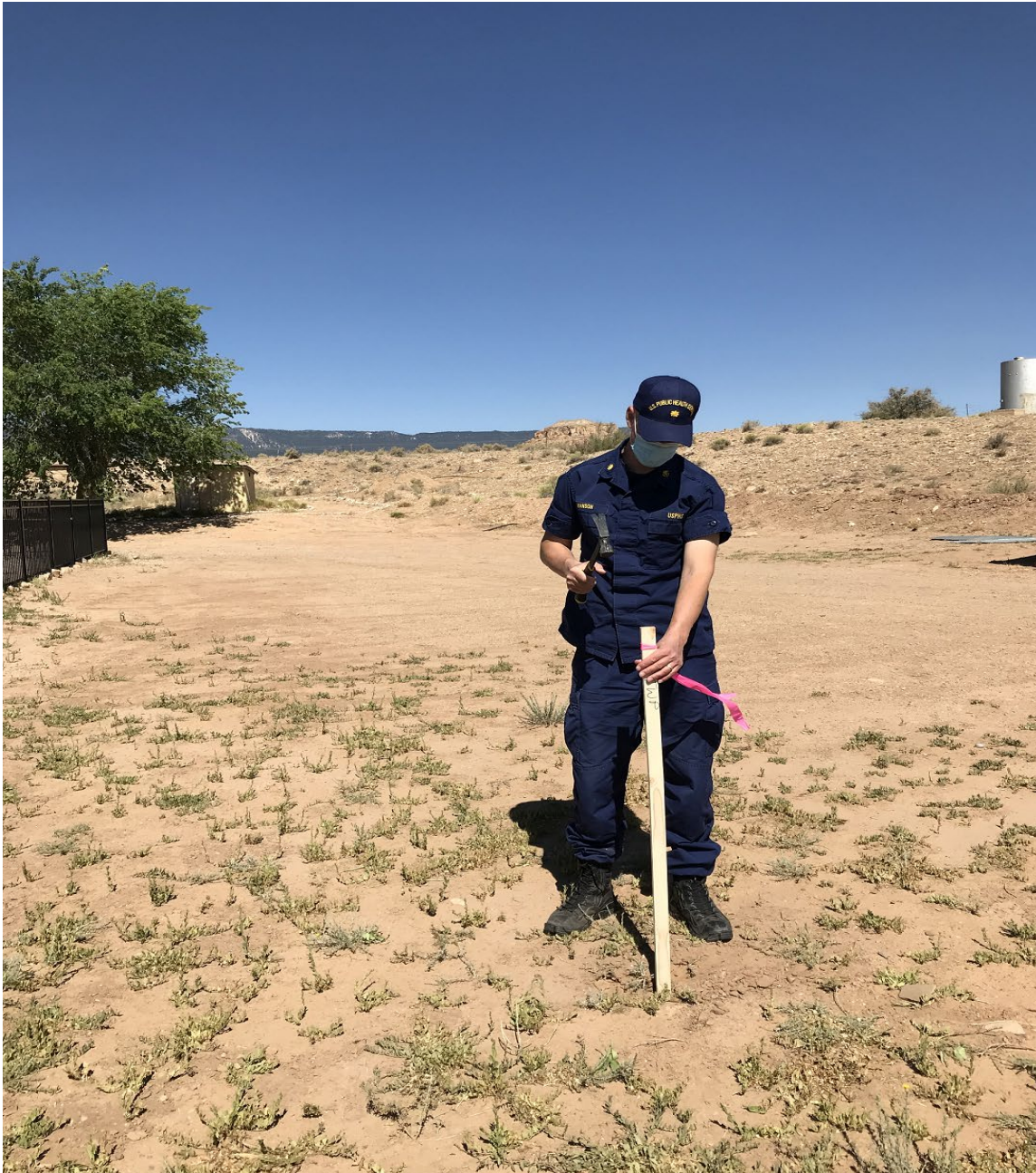
LCDR Hanson installing marker for proposed community watering point, 06/11/2020.
