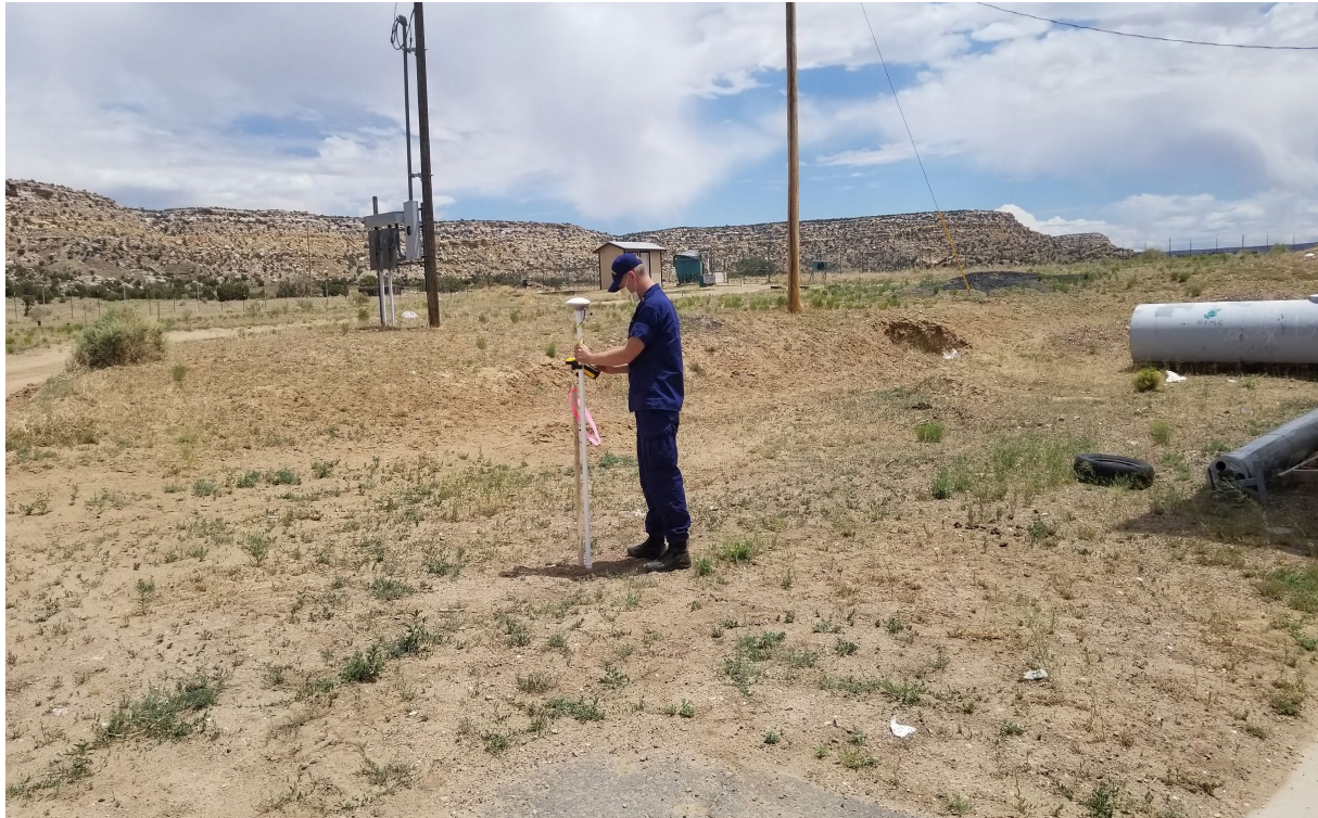
LCDR Hanson surveying a proposed community watering point location 06/03/2020.
