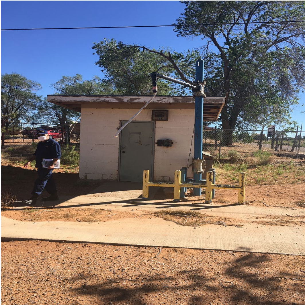
LCDR Ali inspecting existing community watering point facilities, 06/10/2020.
