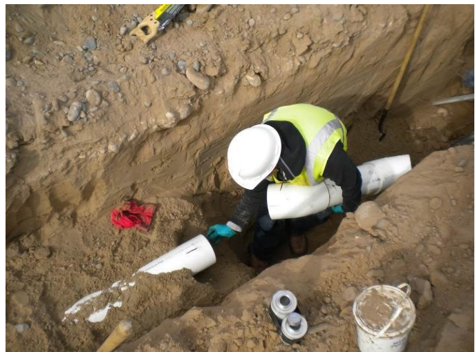
Installing a Sewer Lift
