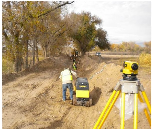
Vacuum Sewer Line Installation
