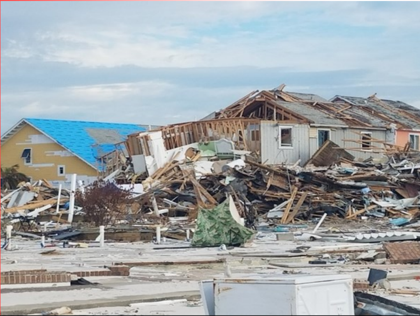
Destruction at Mexico City Beach, Florida.
