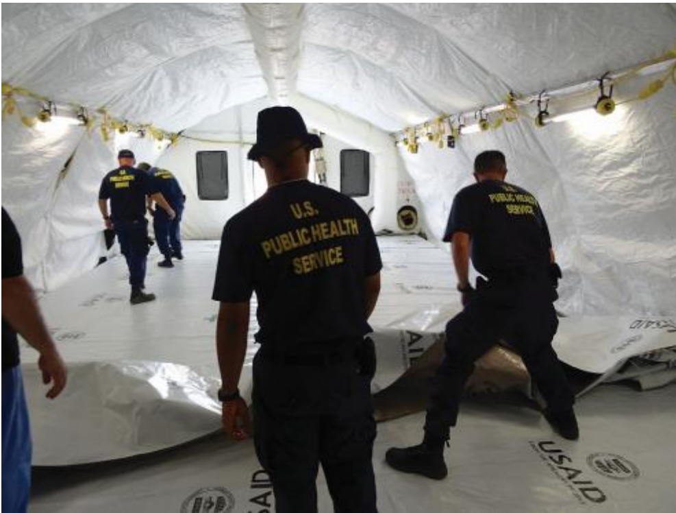
U.S. Public Health Service officers reinforce flooring tarpaulin in the Monrovia Medical Unit's confirmed ward. The medical facility was constructed to care for medical workers who became sick while treating Ebola patients. U.S. PUBLIC HEALTH SERVICE PHOTO
