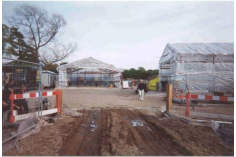
Temporary structures at the Cumbria field office for end-of-the day disinfection of vehicles and equipment (rubber boots, rain suits, etc.).
