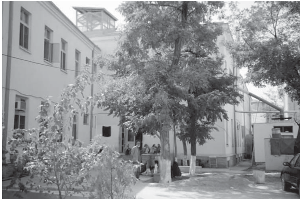
This is the front entrance to the Rabia Balkhi Hospital in Kabul. The HHS OB/GYN project is housed in this hospital.
